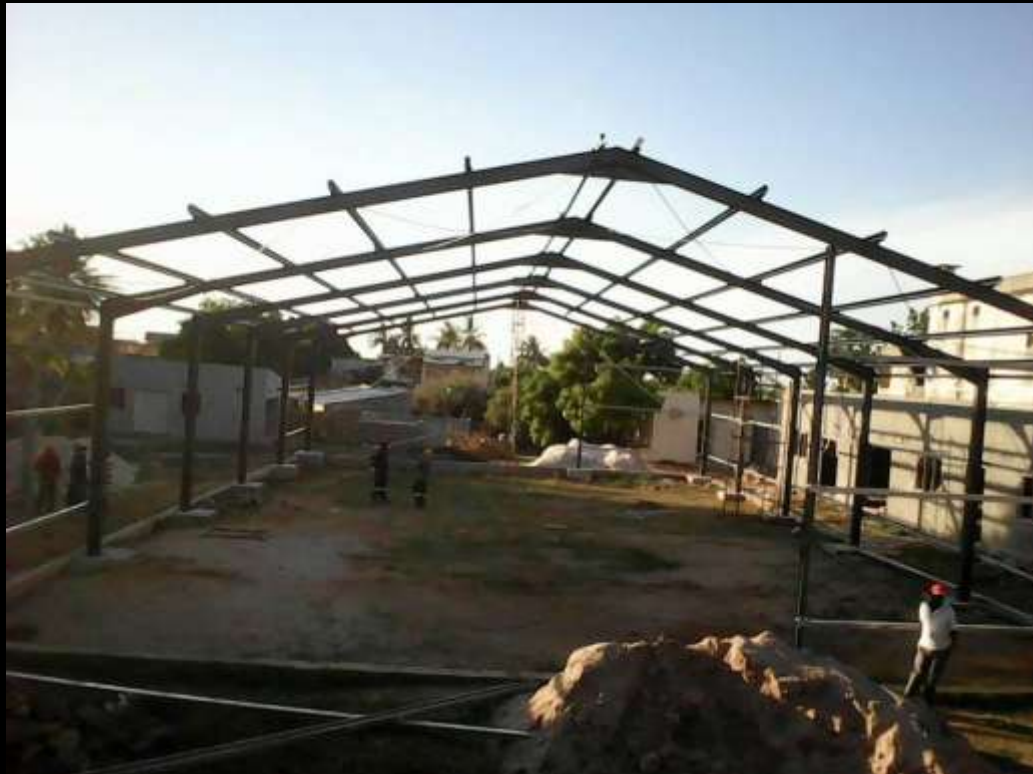
Steel frame erection November '16
